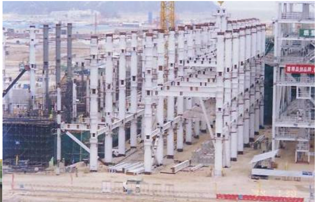
Lanxi Power Plant (China) Cross-columns and heavy sections in HISTAR460
